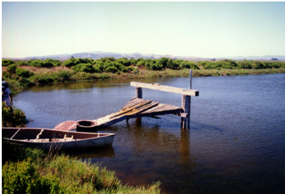
Notice the access shaft to the siphon just behind the canoe. Instrumentation was fixed to these platforms where possible.
